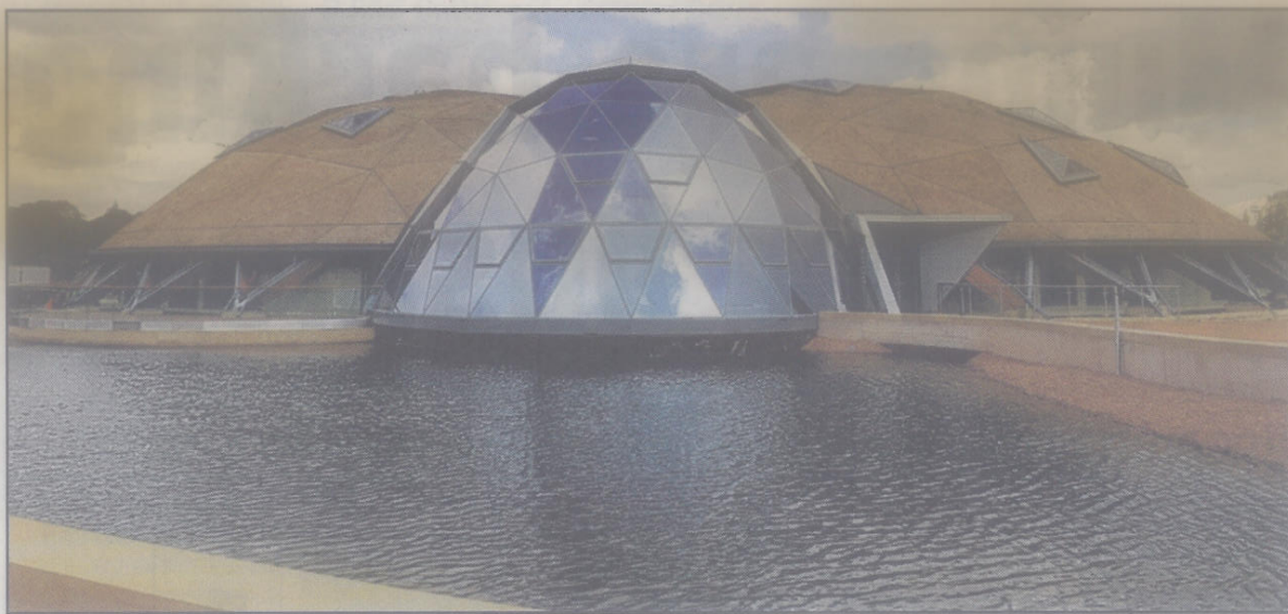
ON SCHEDULE: The Pods leisure centre which will open on Monday.
